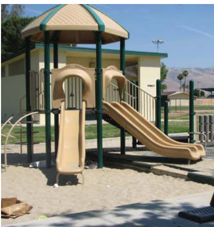
Play equipment in DiGeorgio Park showing need for maintenance and repair
