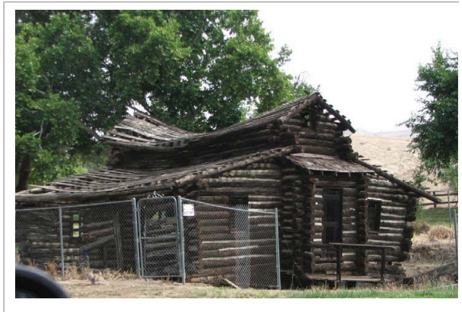
Waterwheel building in Hart Memorial Park
